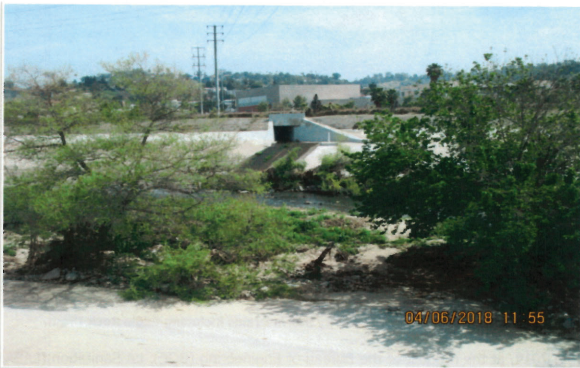
Figure 2: View from West Bank of LA River, Looking Across to Eagle Rock Drain RCB and Outfall Showing Dry Weather Flow. Taylor Yard G2 Parcel is Above and Behind Outfall.
