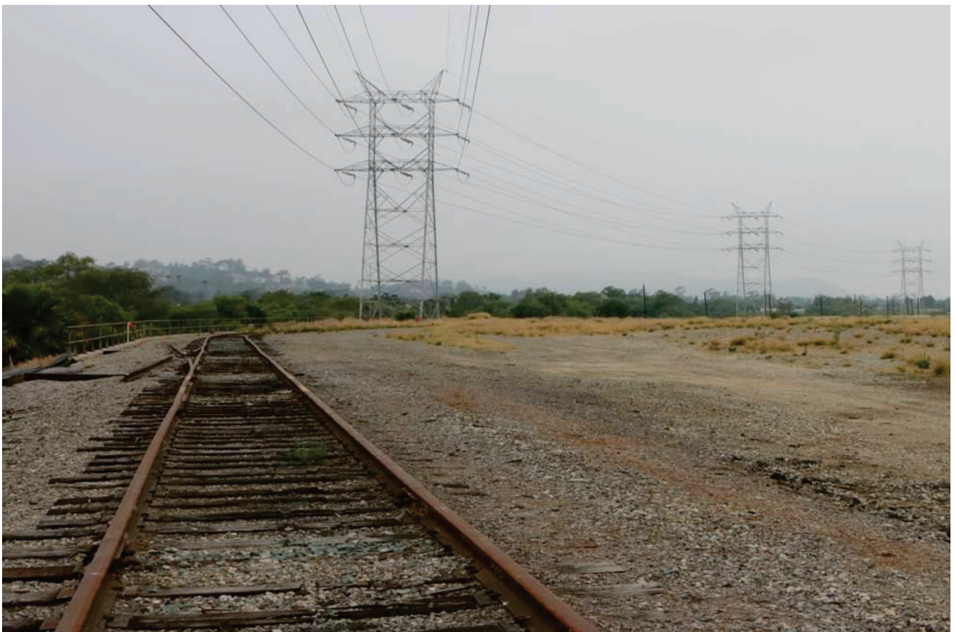
Figure 4-1. Picture of Existing Power Lines at the Project Site
